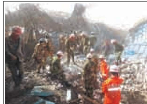
Rescuers work at the accident site of a collapsed building in the Da Qaidam (also known as Dachaidan) district in the Mongolian-Tibetan Autonomous Prefecture of Haixi, northwest China's Qinghai Province, on 12 Oct, 2013. Five people have been buried and 16 others injured when the building collapsed Saturday afternoon, and the buried were confirmed dead during the ongoing search. — XINHUA
