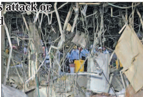
A view of the inside of the headquarters of state-owned oil giant Pemex in Mexico City on 1 Feb, 2013.—REUTERS
