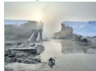
Photo taken on 2 Feb, 2013 shows the breached dyke of the Lianfeng Reservoir in Urumqi, capital of northwest China's Xinjiang Uygur Autonomous Region. XINHUA
