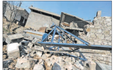
Photo taken on 1 Feb, 2013 shows the cracked and collapsed houses at Zhongtun Township in Zhenxiong County, southwest China's Yunnan Province. A landslide destroyed 35 houses, damaged 928 others and affected the lives of 712 people here. All villagers who were affected by the landslide have been relocated, the county government said. No casualties have been reported.—XINHUA
