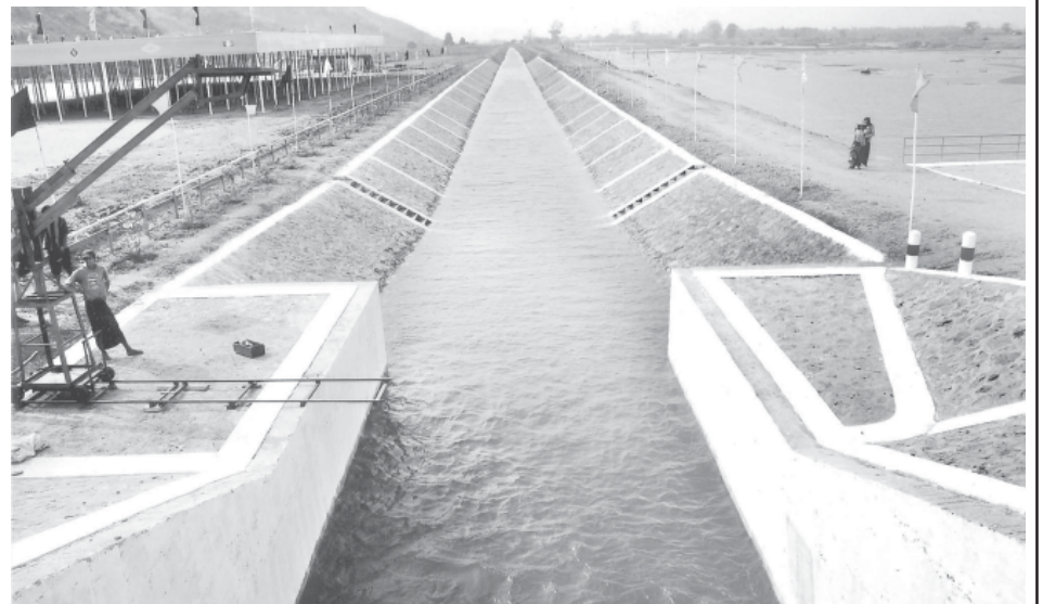
Water flowing in 29.72 miles long left main canal of Paunglaung Diversion Weir to irrigate 16,000 acres of farmlands.
