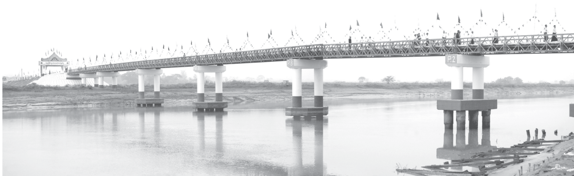
Newly built Bago River Bridge (Kawa).—MNA
