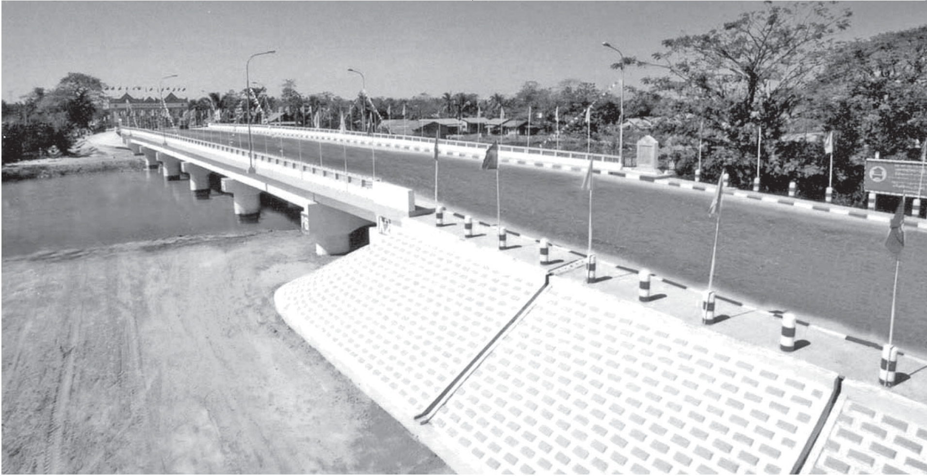
Yenwe Chaung Bridge in Nyaunglebin Township.
