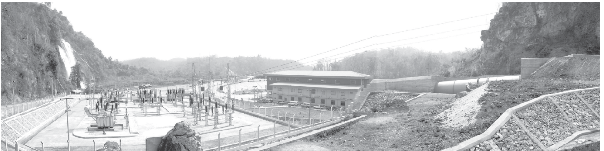
Kengtawng Hydropower Station with Kengtawng Falls.—MNA
