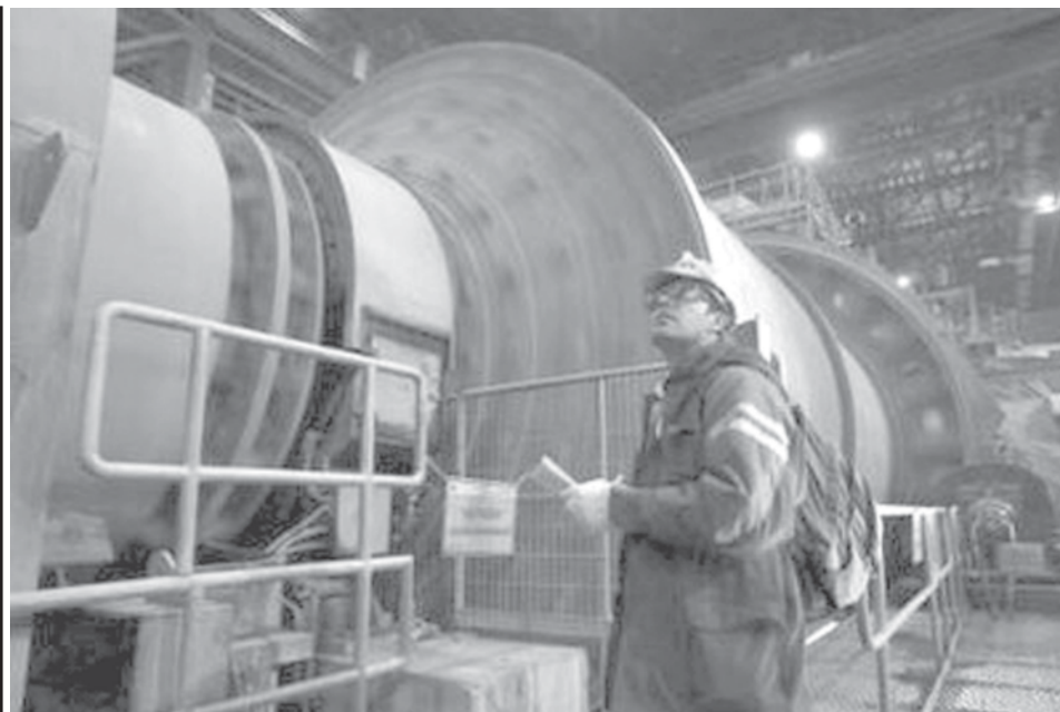
Reuters' correspondent Simon Gardner looks inside the copper mills building at the Los Bronces copper mine, about 60 km (40 miles) northeast of Santiago and 3500 metres above sea level, on 20 March, 2009.—INTERNET
