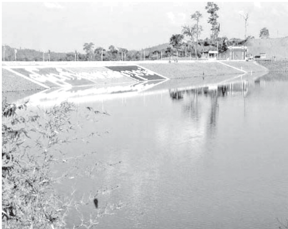
Photo shows water being stored at North Yama Supporting Dam in Pale Township of Monywa District, Sagaing Division.
