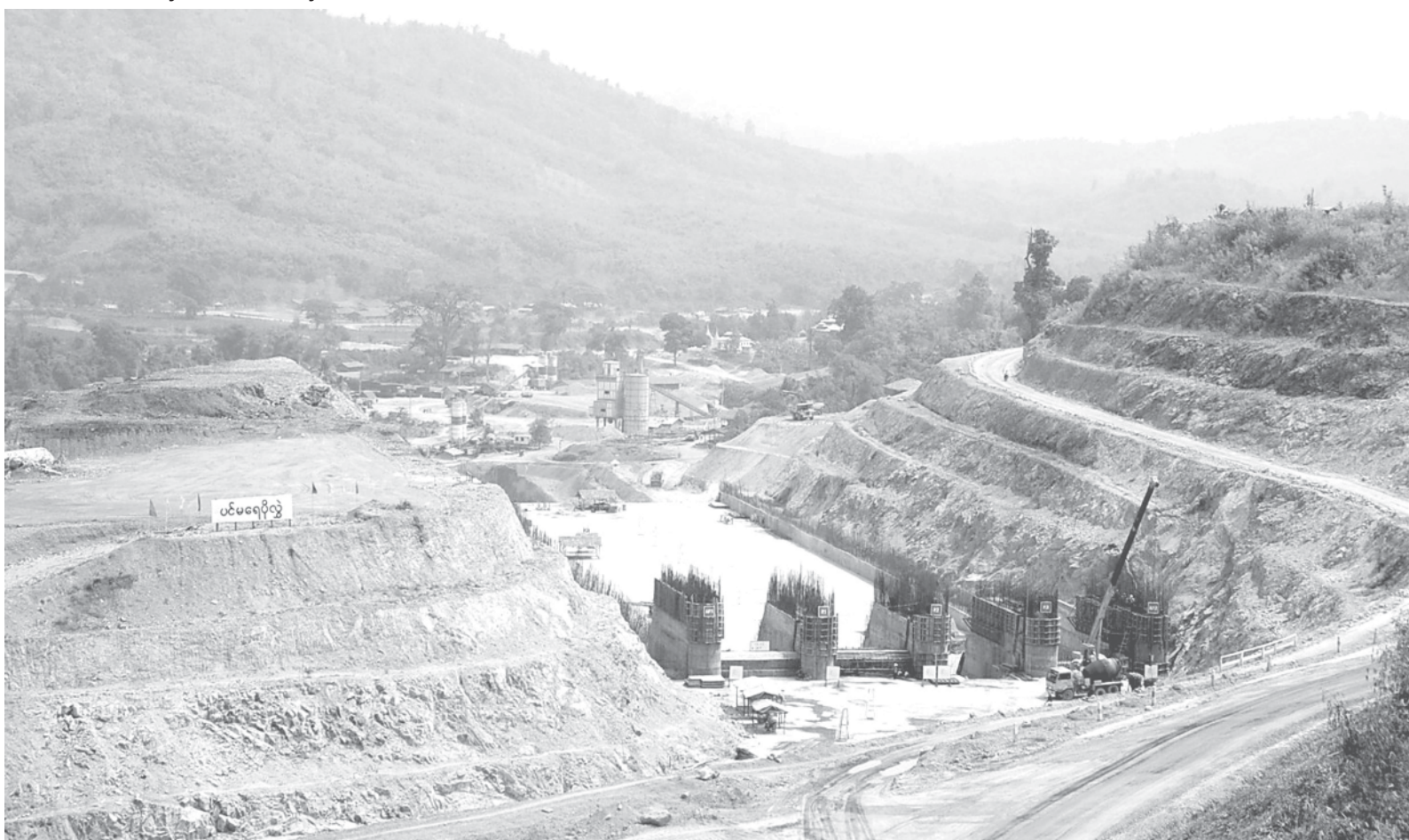
Photo shows progress in implementing the Shwegyin hydropower plant project.—MNA
