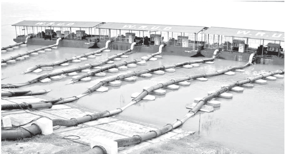
River water pumping projects benefit arid region Sagaing Division to be able to grow summer and monsoon paddy.
