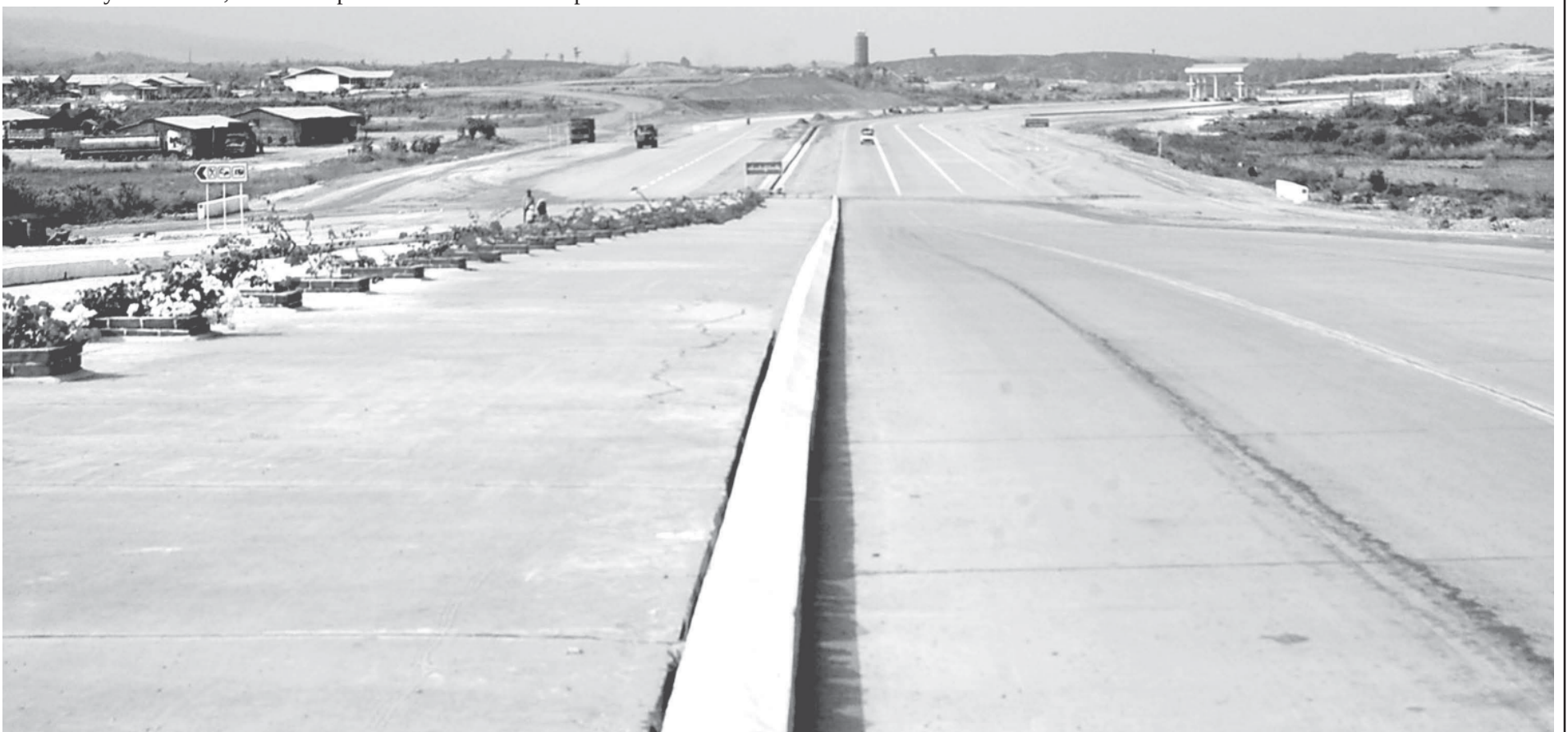
Tatmadawmen are also participating with might and main in building Yangon-Mandalay Expressway. Its Nay Pyi Taw-Yangon section will be opened soon.
