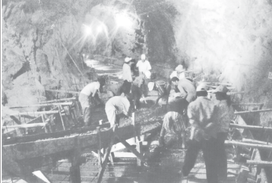
Engineers and skilled workers constructing water intake tunnel.
