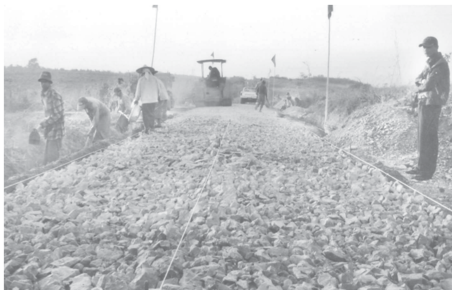
Gravel being placed on Pyinsar-Pauktaw inter-village road.
