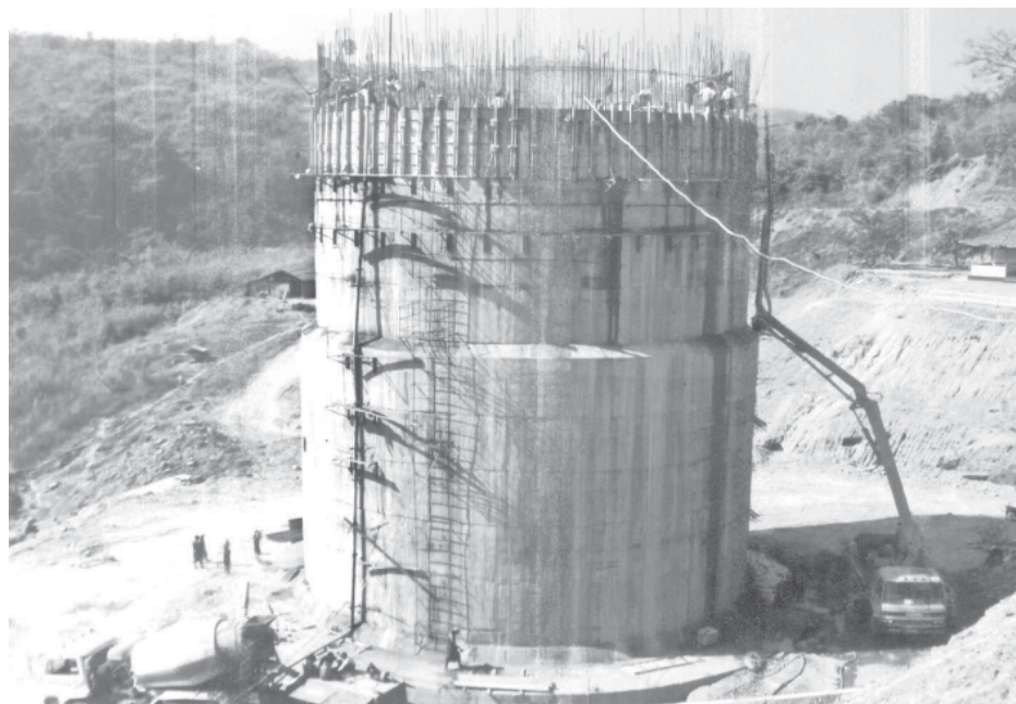
Surge drum is being built at Kunchaung Hydropower Plant.
