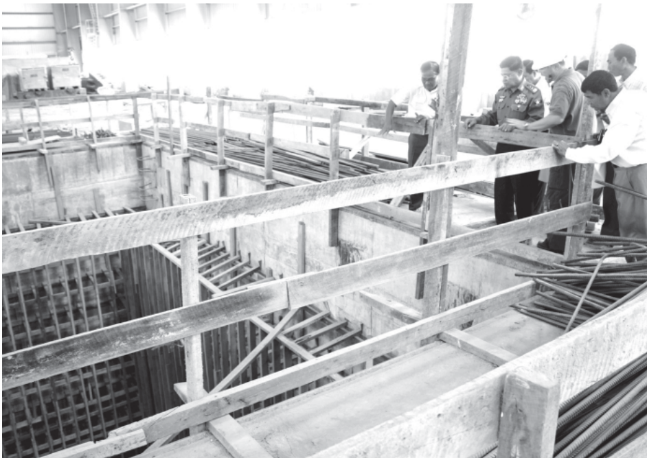
Industry-2 Minister Vice-Admiral Soe Thein inspects completion of machine foundation of 16-ton Press Machine at Forging Shop.
