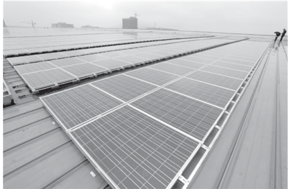
The photo taken on 2 March, 2009 shows a matrix of solar panels in Hefei Solar PV Power Plant, in Hefei, capital of east China's Anhui Province. The Solar PV Plant built by Hefei Sunshine Power was combined to the state power grid 1 March with a total installation capacity of 500 kilowatts and annual capacity of 600,000 kilowatt-hours.—XINHUA
