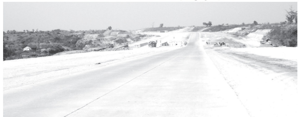
Photo shows already-built Myochaung-Tagara road section at mile post (119/0). —MNA
