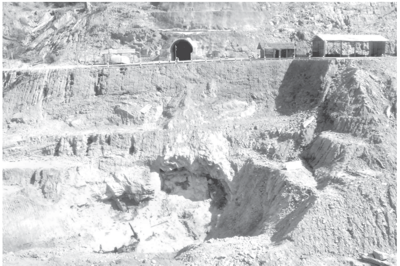
Photo shows land preparations at Salu Creek for building concrete posts of the bridge for intake tunnel and aqueduct.
