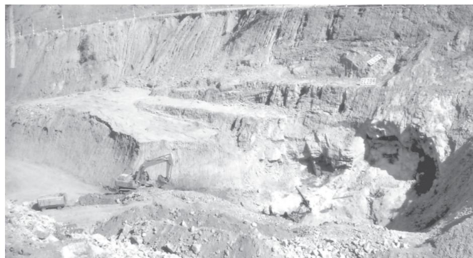
Ground preparations being made for construction of concrete posts at Salu Creek.
