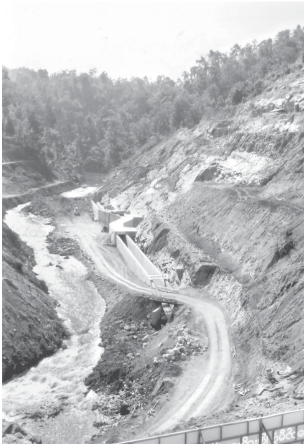
Diversion conduit seen near Nancho Creek.
