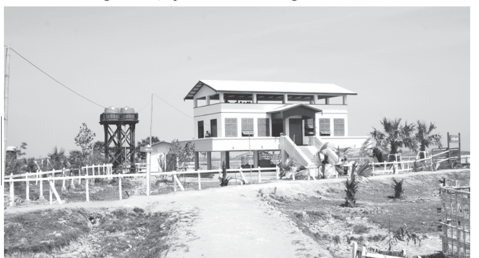
Cyclone Shelter in Auk-pyun-wa village of Labutta Township constructed by FMI Co.—MNA
