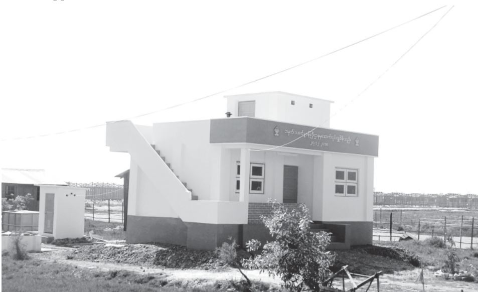
Photo shows the cyclone shelter built by Industry-1 Ministry in Pyinsalu.—MNA
