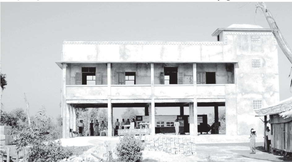
Cyclone Shelter in Kanhtu Kantha ward of Pyin Khayaing in Labutta Township donated by Mitta Development Foundation.—MNA
