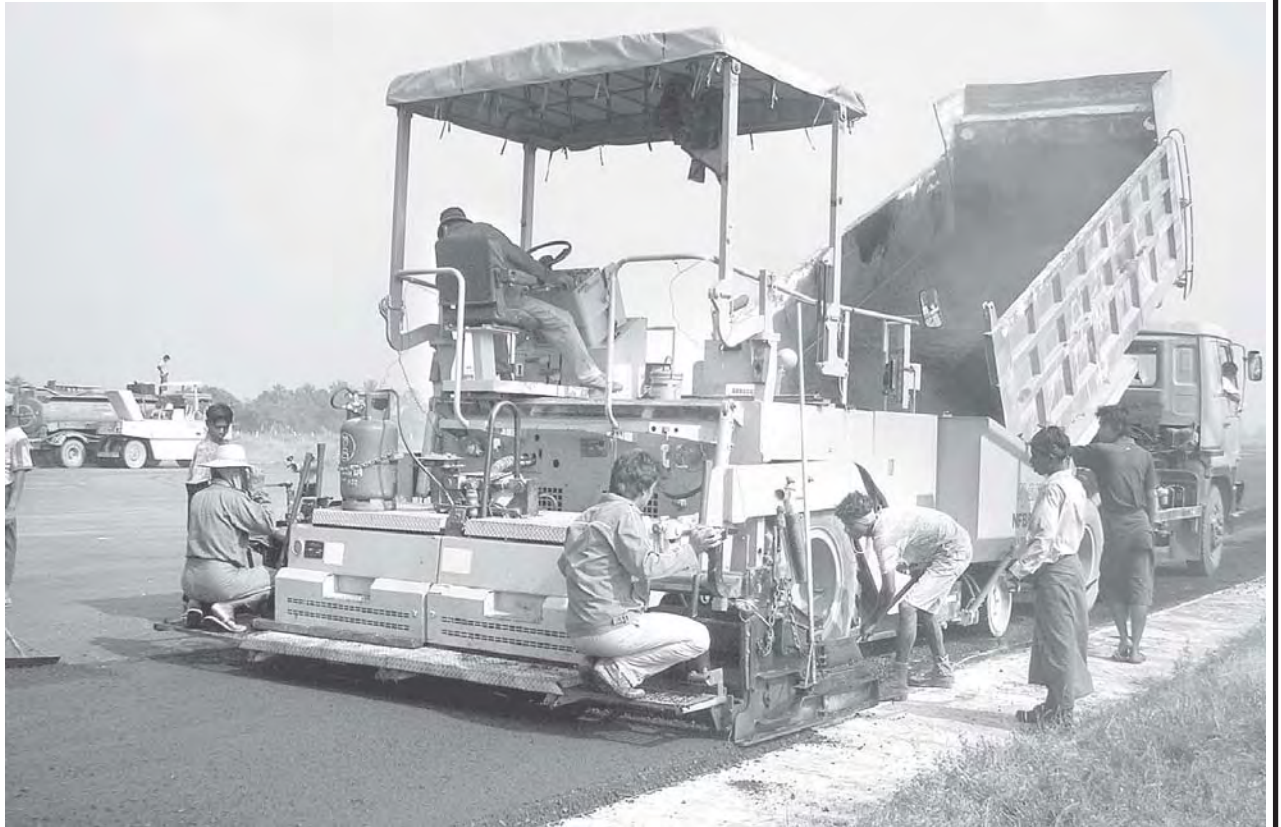
Workers resurfacing the runway.
