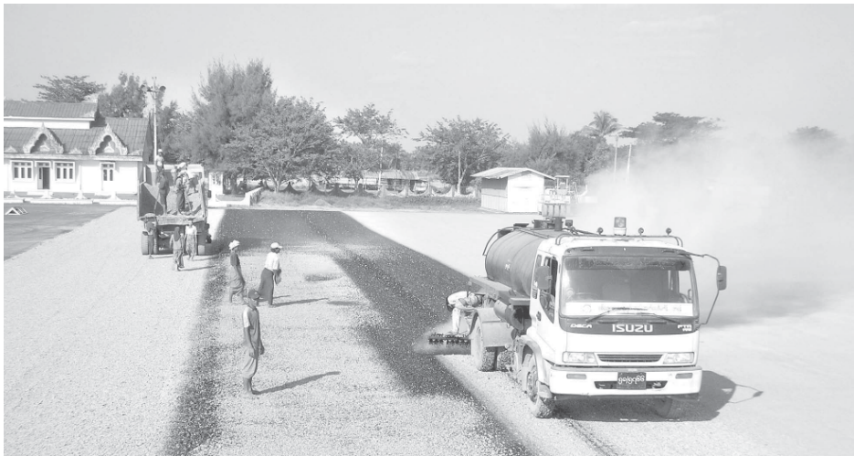
The tarring of the runway in progress.
