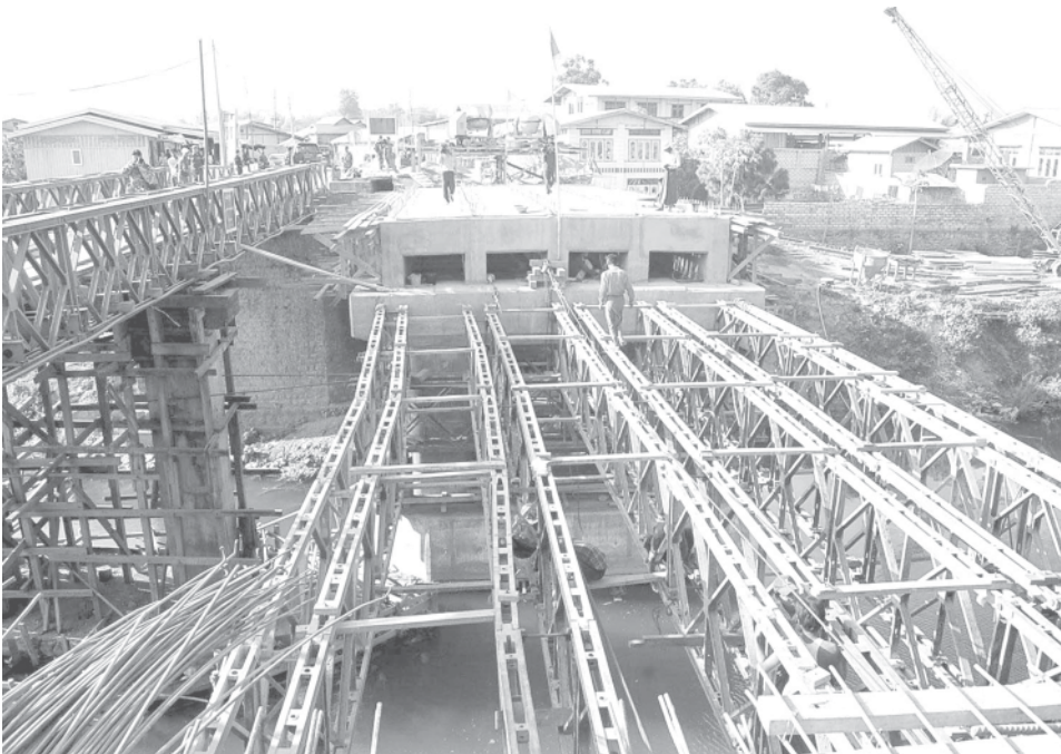
Implementing of Nampaung Bridge project in progress.
