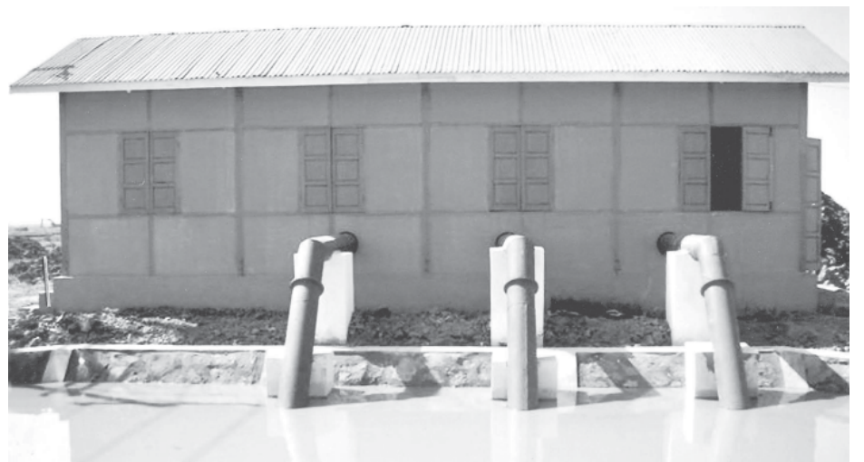
Sitpin river-water pumping station in Hlegu Township.
