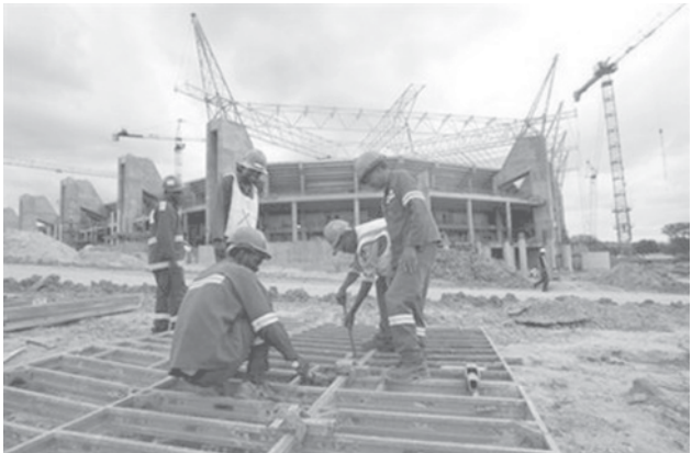
Labourers work at the site of Nelspruit's new football stadium, set to be one of the ten stadia across South Africa used during the 2010 World Cup, on 19 January. The 2010 World Cup to be hosted by South Africa will leave the legacy of security in the country and of pride on the continent, FIFA president Sepp Blatter said on Monday. —INTERNET
