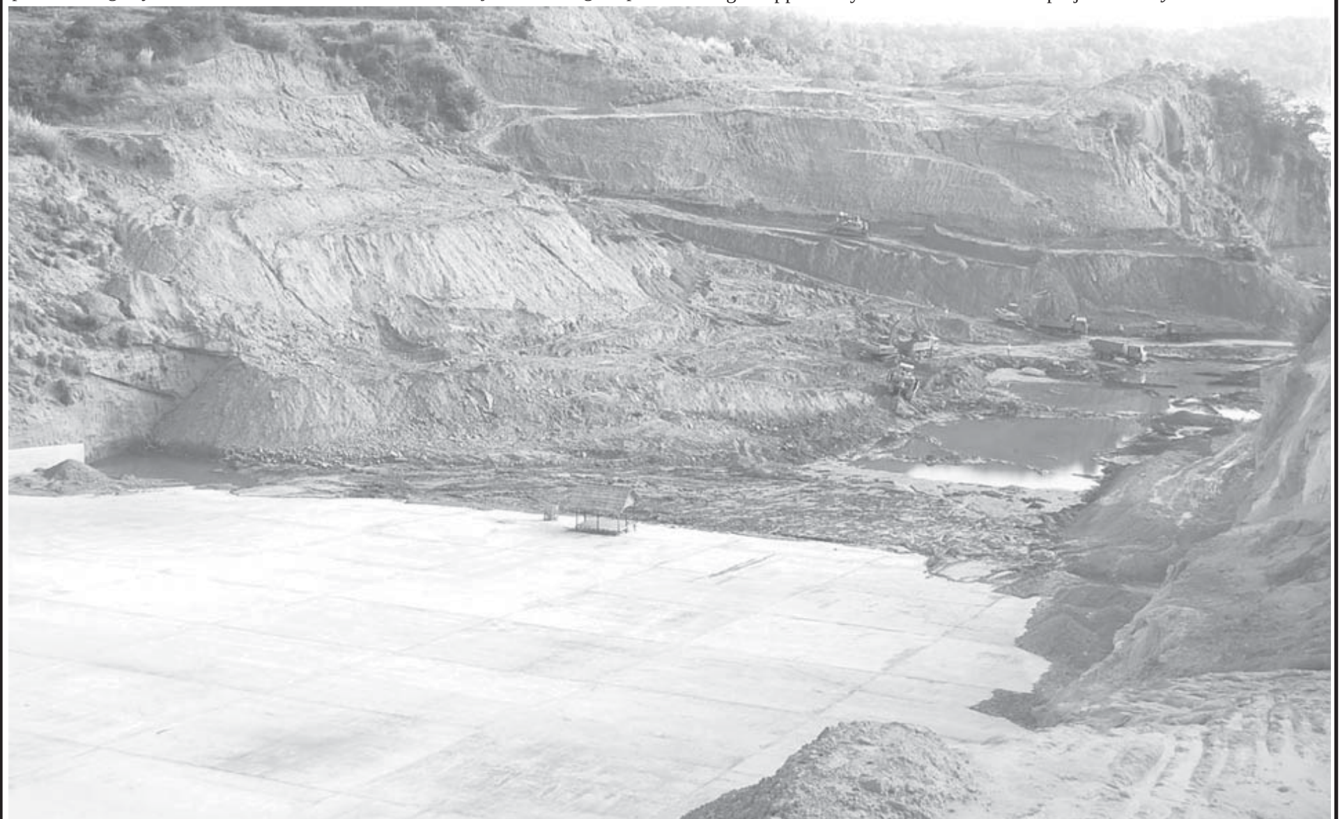
Kyeeohn-kyeewa Dam is under construction near Wunlo Village of Pwintbyu Township on 5 November 2008.
