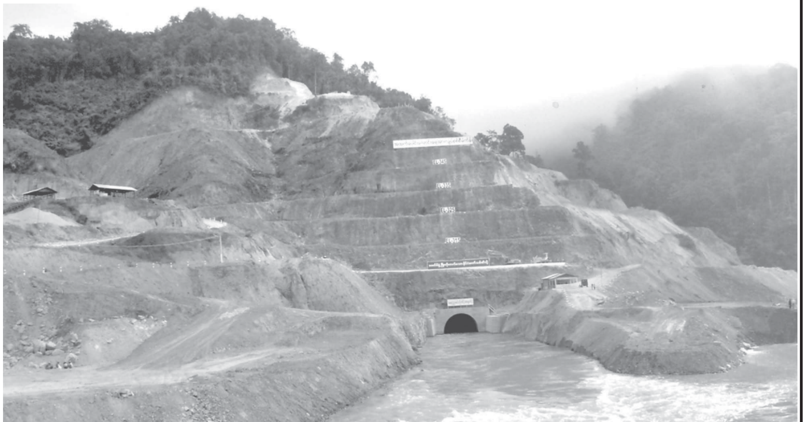
The diversion tunnel of Upper Paunglaung Hydropower Project.
