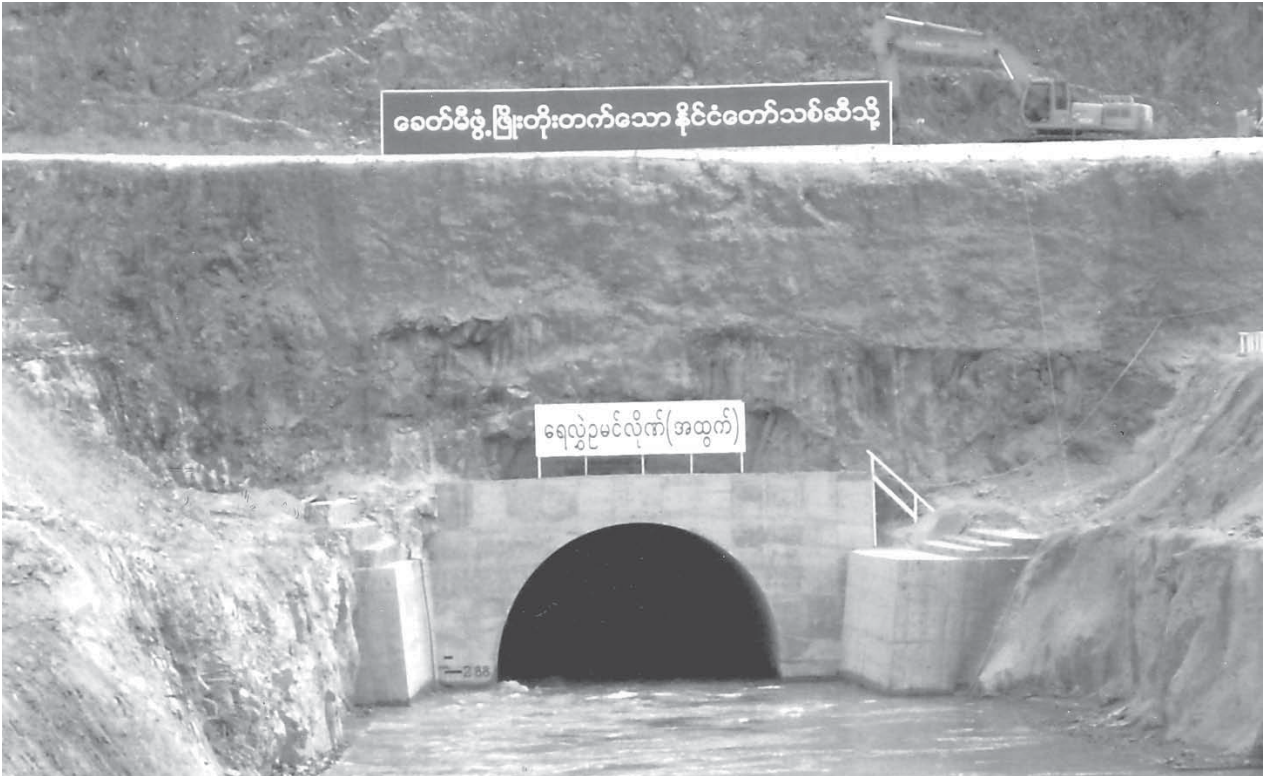
The outlet portal of the diversion tunnel of Upper Paunglaung Hydropower Project.
