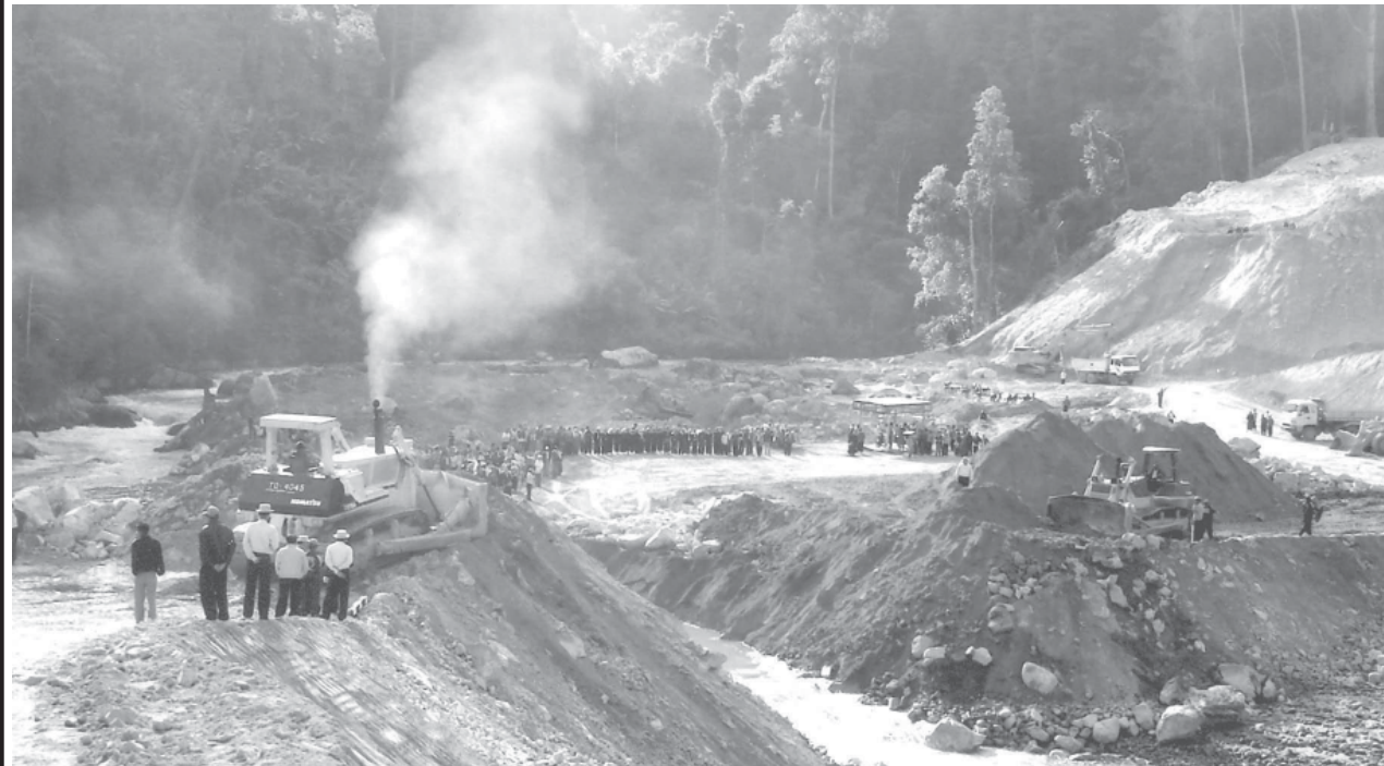
The Paunglaung River was blocked on 5 December 2008 to divert its current.
