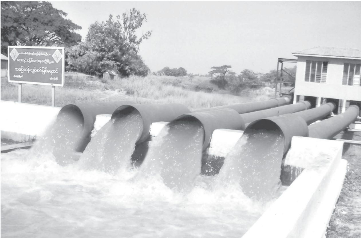
Thabyetan river water pumping station supplying water from Hline River to farmlands through main canal.
