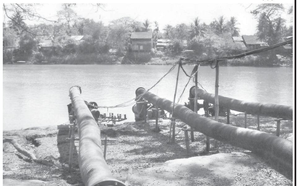
Taungyat Zigon river water pumping station installed with water pump and pipes to use water from Hline River.
