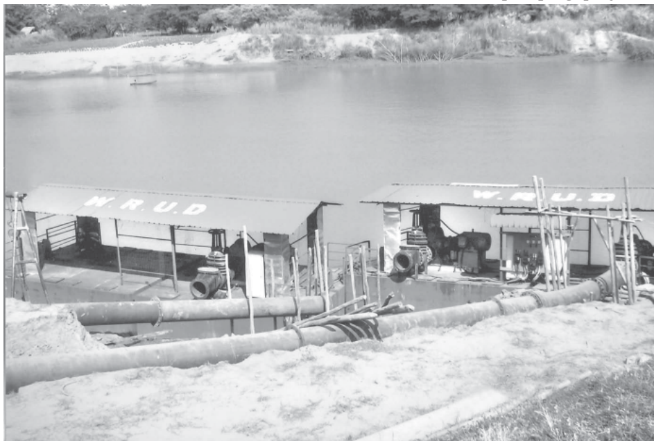
Aingkalaung river water pumping station pumping up water from Hline River by water pump and pipes.
