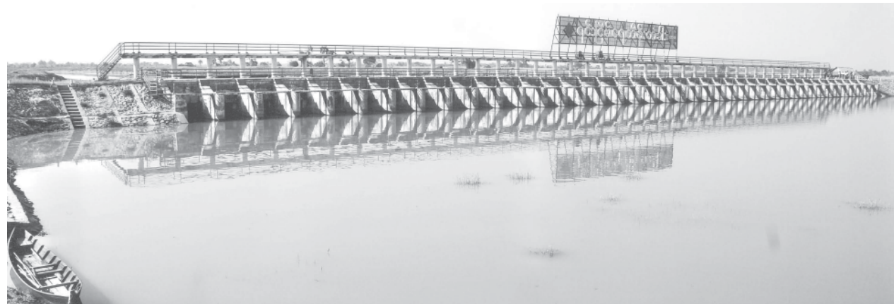
Yinnyein Sluice Gate built with 40 valves in Kyonhtaw Village of Paung Township to control the inflow of sea water and supply of fresh water.
