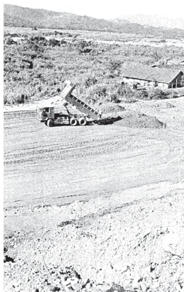
A truck at the project site.
