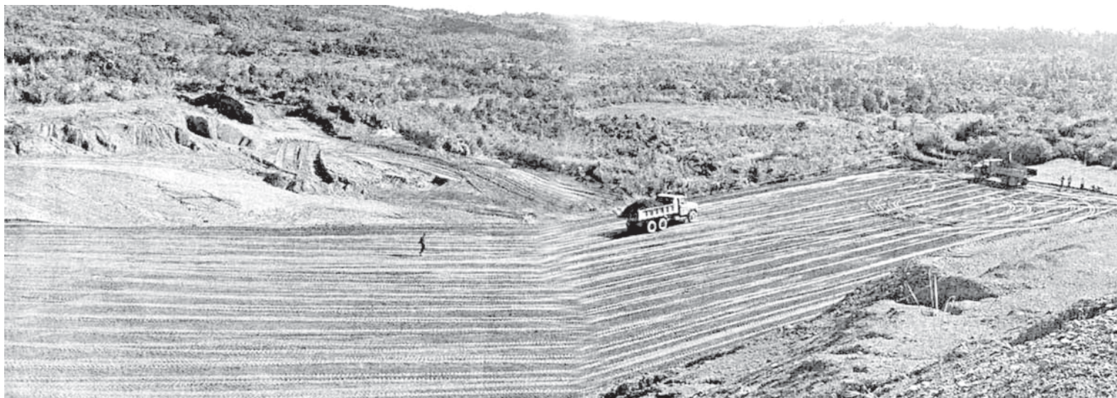
An aerial view of the construction site.
