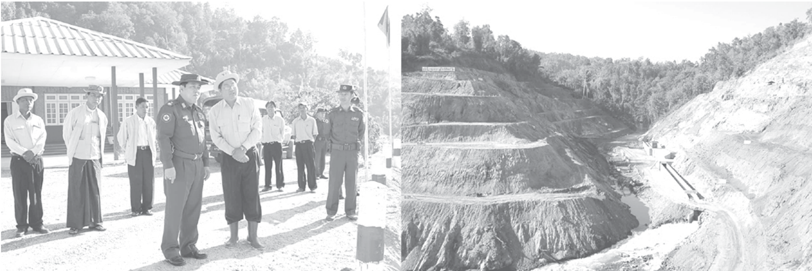
Commander Maj-Gen Wai Lwin inspects construction tasks of Nancho Hydropower Project in Nay Pyi Taw Pynmana.—MNA
