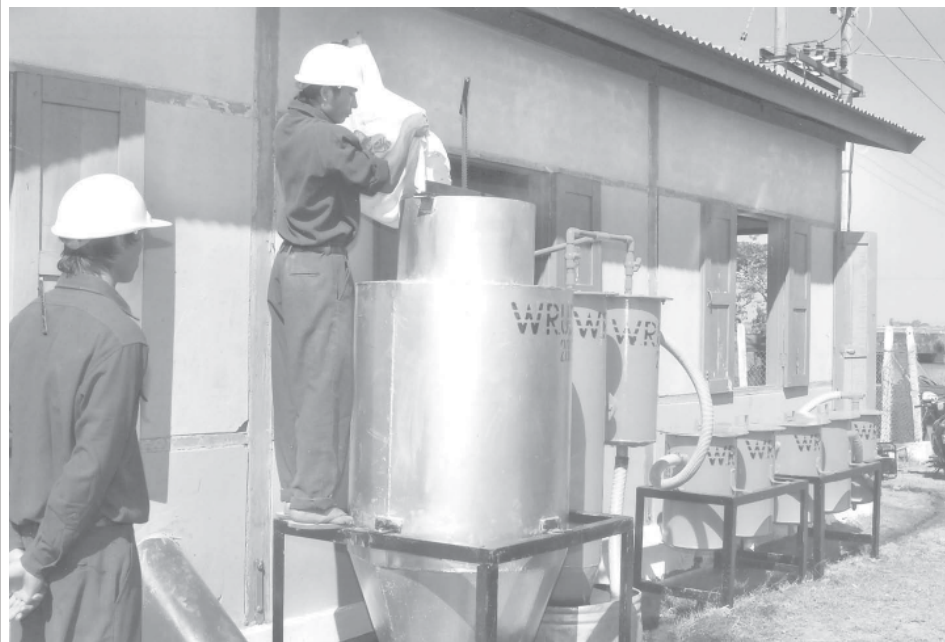
An employee pouring paddy husk into fuel tank at Balar Water Pumping Station.
