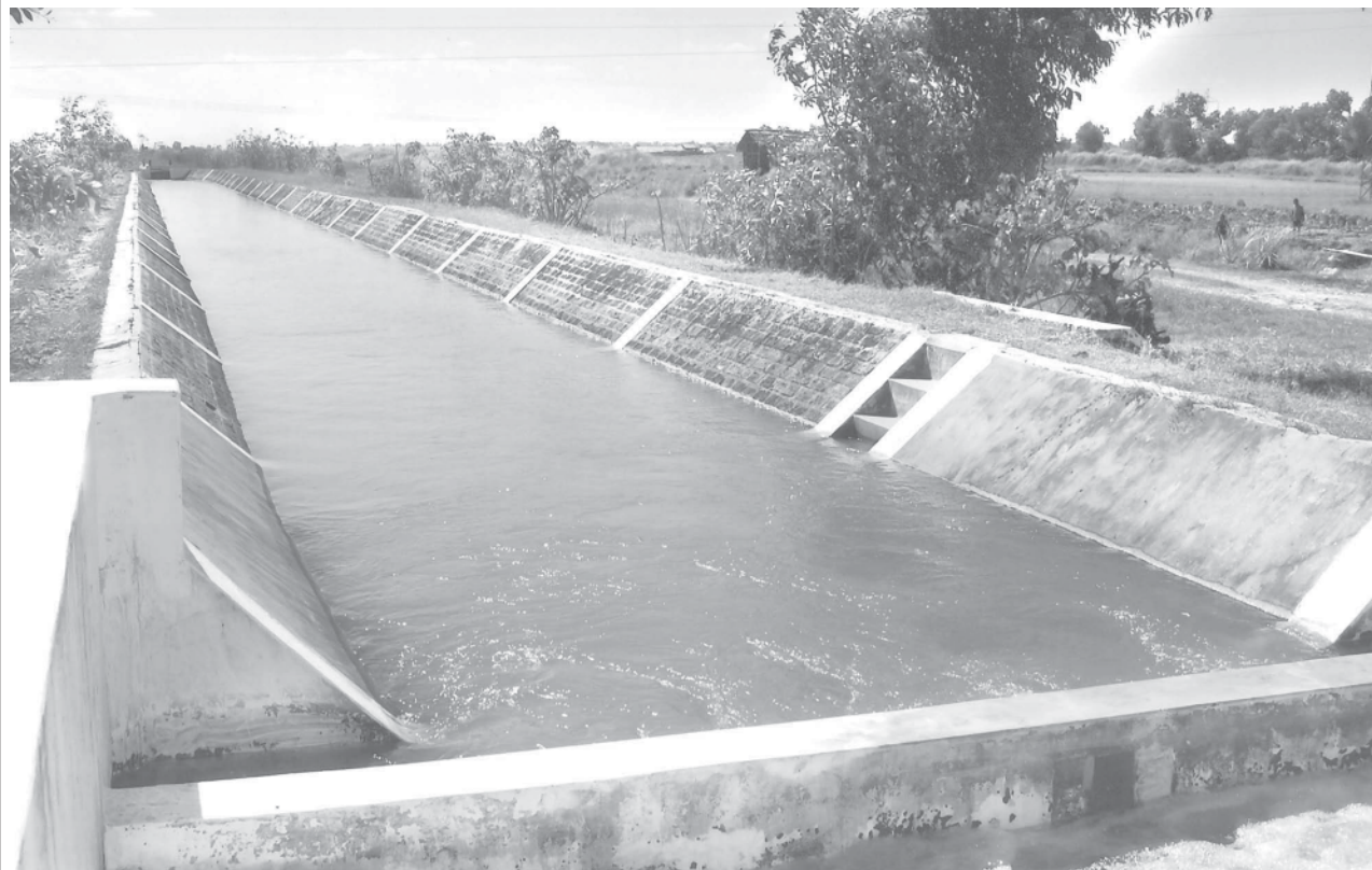
The main canal of Balar Water Pumping Project.
