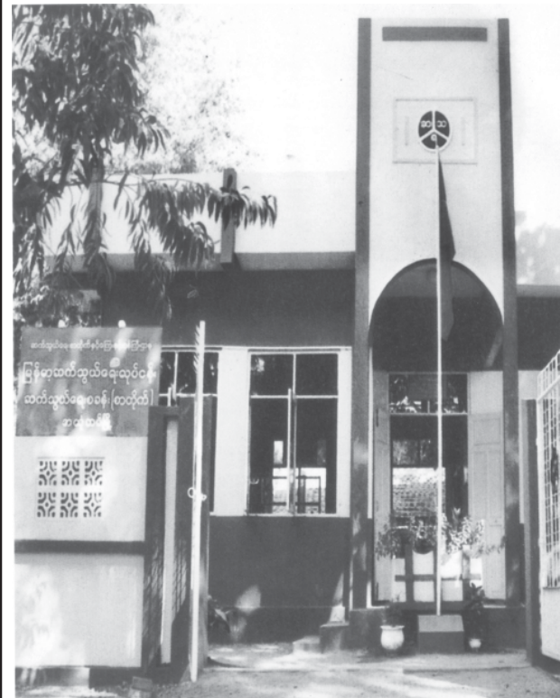
Myanmar Posts and Telecommunications Centre constructed in Ahlon of Monywa Township for enhancement of communications sector.
