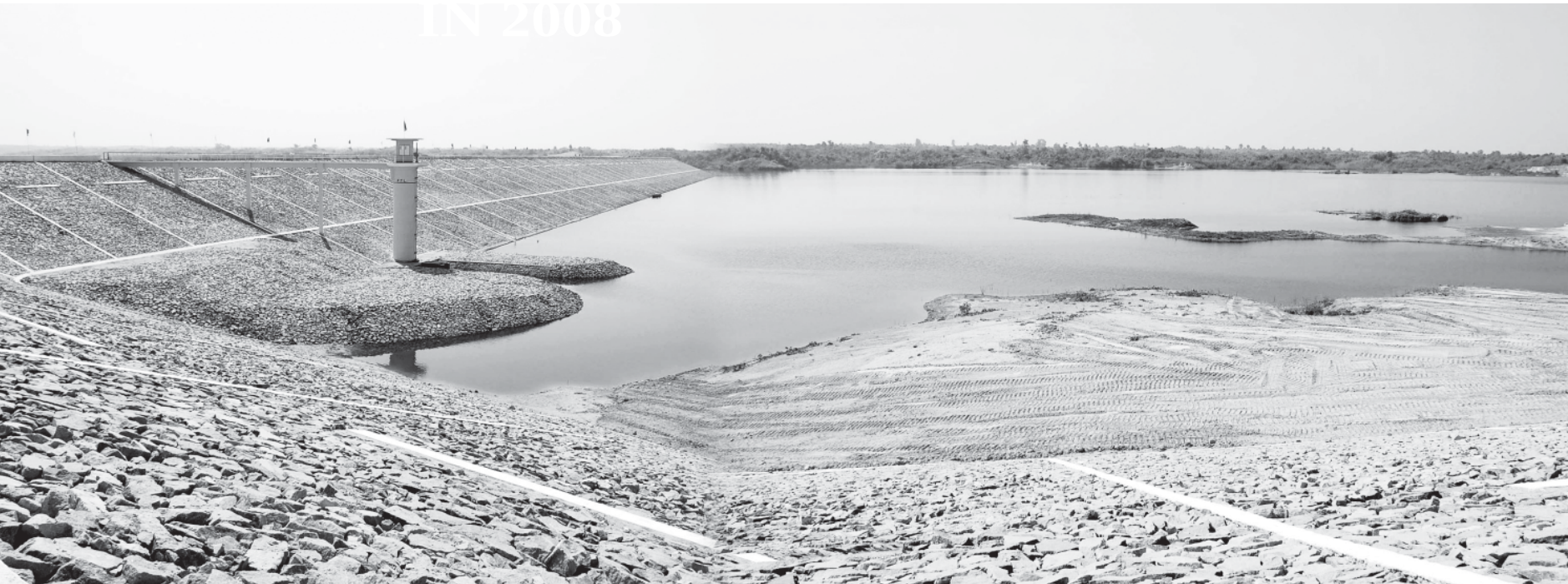
Photo shows Wagadok Supporting Dam opened on 26, January 2008 near Taungsatinn Village, Bago Township.
