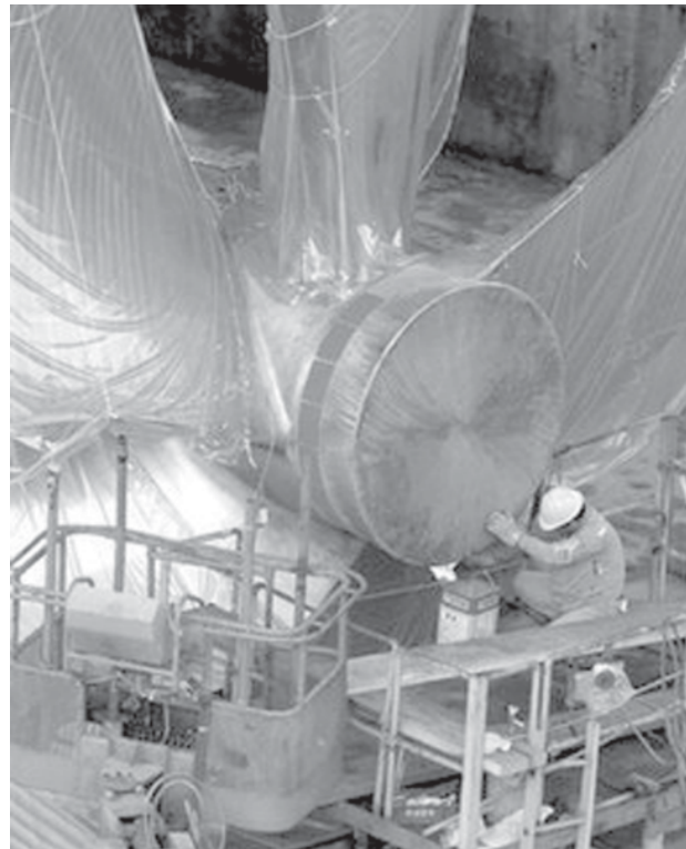
A ship being built at a shipyard in Ulsan, South Korea. South Korea's state-run Korea Development Bank has said it will delay finalising a deal to sell the world's third largest shipyard, Daewoo Shipbuilding and Marine Engineering.—INTERNET
