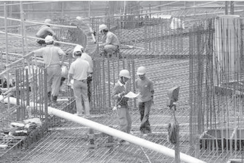
Work takes place at a construction site of a residential development in Singapore on 23 Sept, 2008. Singapore’s annual inflation stood at 6.4 percent in August, slightly higher than expected, because of rising food and housing costs but falling further from a 26-year high.—INTERNET
