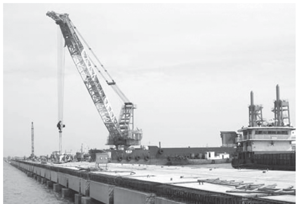
The mother harbour for international liners is seen under intense construction to the southern end of Dongjiang Bonded Harbor Area in north China's Tianjin Municipality, on 10 Sept, 2008. The first phase of the harbor area includes two container terminals and warehouses along with a 625-meter-long coastline and it can harbor the present largest liner in the world with a designed annual passenger capacity of over 500, 000 person-time.—XINHUA
