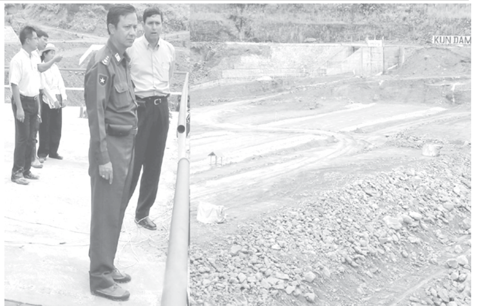
Minister Col Zaw Min inspects earth work of Kunchaung Hydropower Project. — MNA
