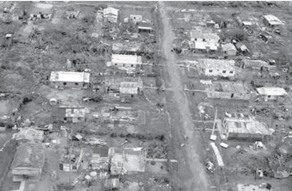
Houses destroyed by Hurricane Ike stand in Pinar del Rio on 11 September, 2008. Ike has caused widespread damage and a panorama of destruction in Cuba, still reeling from the more powerful Hurricane Gustav 10 days ago.—INTERNET
