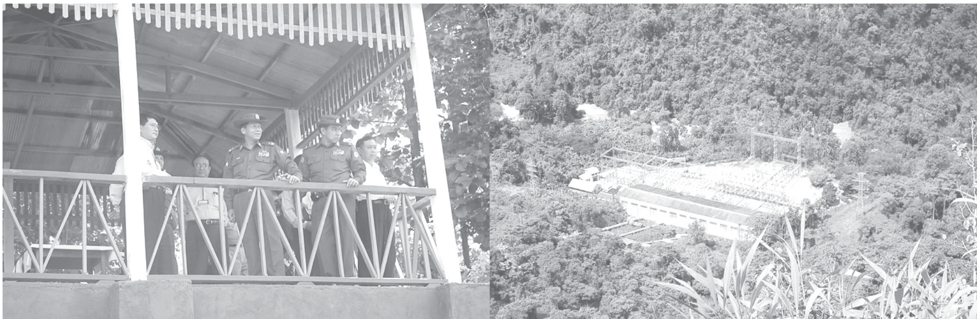
Maj-Gen Min Aung Hlaing inspects No. 2 Beluchaung Hydropower Plant (Lawpita) in Loikaw Township.—MNA
