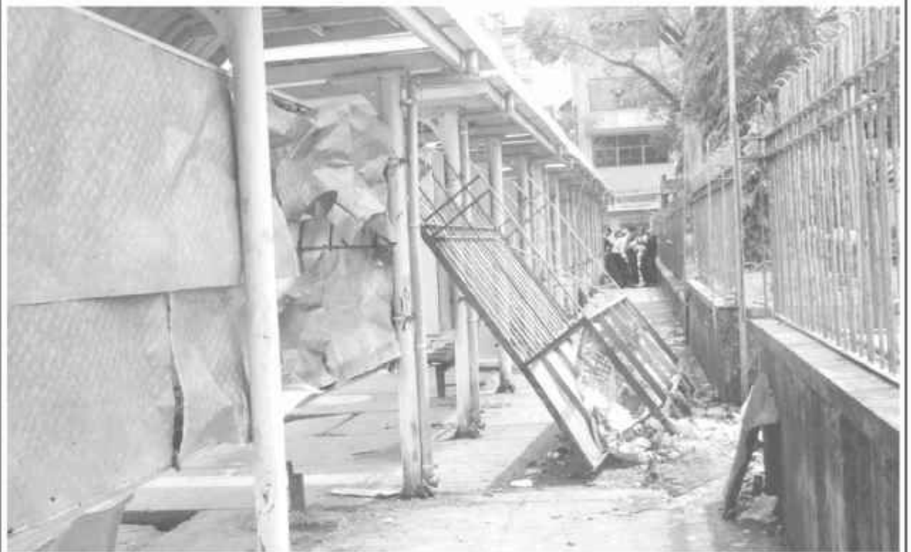
Damage caused by bomb blast at Maha Bandoola Park. —MNA
