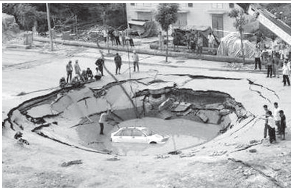
A stranded car is hoisted from a collapsed road surface in Guangzhou, Guangdong Province, on 7 September, 2008. The road collapsed on Sunday afternoon and trapped the car in a hole, which measured 5 metres (16.4 feet) in depth and 15 metres (49.2 feet) in diameter, local media reported. Further investigation is underway. INTERNET
