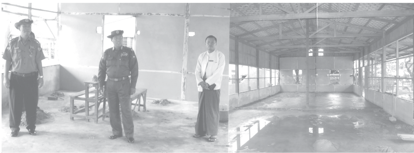
Commander Brig-Gen Tin Ngwe inspects construction of new building for BEPS No. 34 in Mahaaungmyay Township.—MNA
