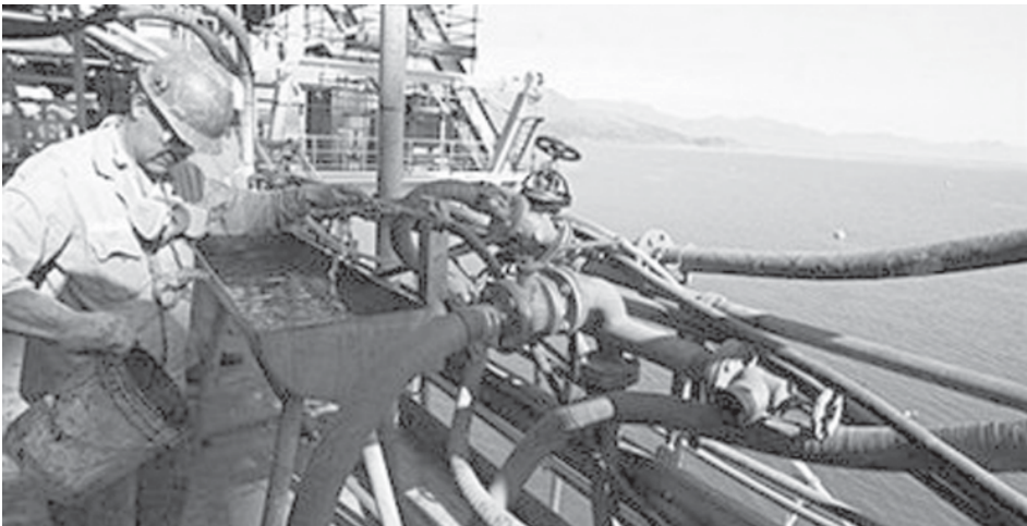
A worker on a deck of an off-shore oil platform construction site in Brazil, in August 2008. Brazil will on Tuesday start to tap a deepwater offshore oil field that could presage how difficult it will be to pump reserves in vast new fields located even farther out to sea.—INTERNET
