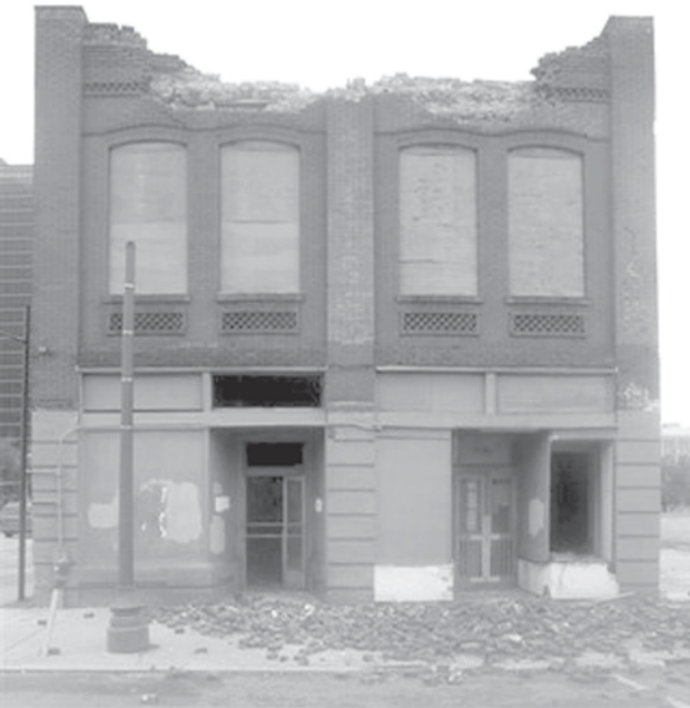
The top of a building lies in the street after being taken down by the winds of Hurricane Gustav in downtown New Orleans, on 1 Sept, 2008.—INTERNET
