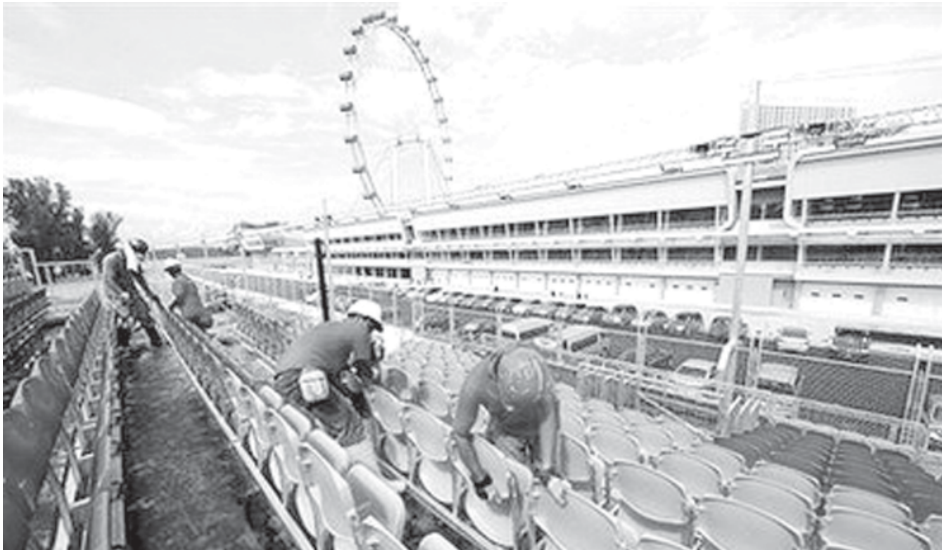
Workers put the final touches on seats in front of the completed three-storey pit building in Singapore recently. Singapore is giving workers in the tourism sector a tune-up before tens of thousands of auto racing fans descend on the city-state for the world’s first Formula One Grand Prix night race.—INTERNET
