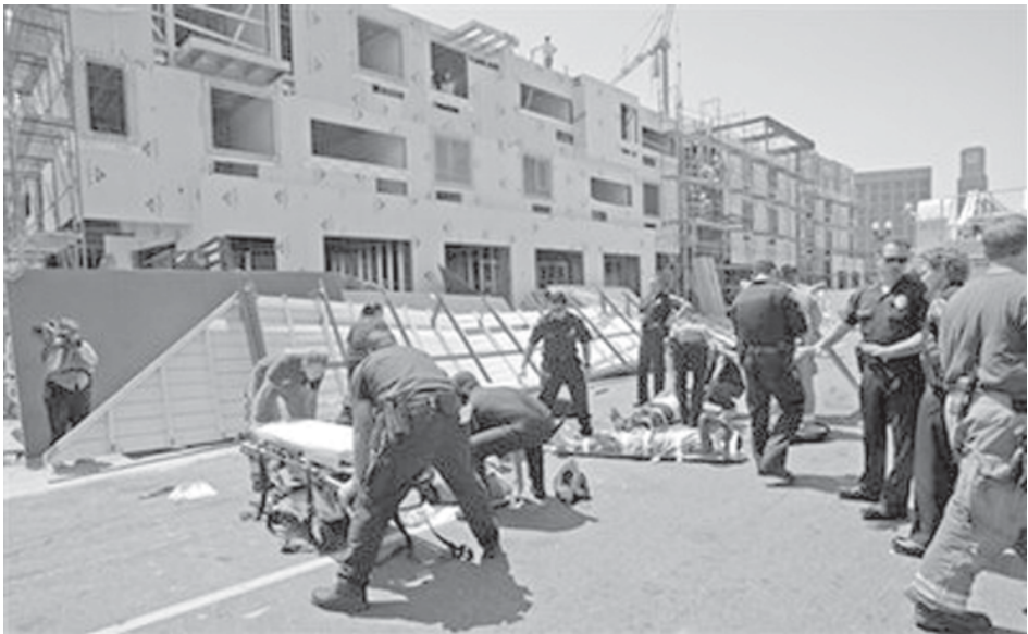
Paramedics, police, and firefighters attend to the injured as construction workers look down from their project where a construction site covered walkway collapsed, injuring at least 16 pedestrians in downtown San Diego on 28 Aug, 2008.—INTERNET
