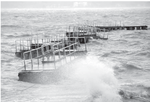
A float bridge is damaged by the gale at Dayawan sea area in Shenzhen, south China's Guangdong Province, 22 Aug, 2008. —INTERNET
