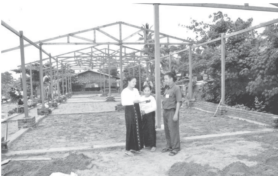
New school building is under construction with steel structure and without timber for its durability.
