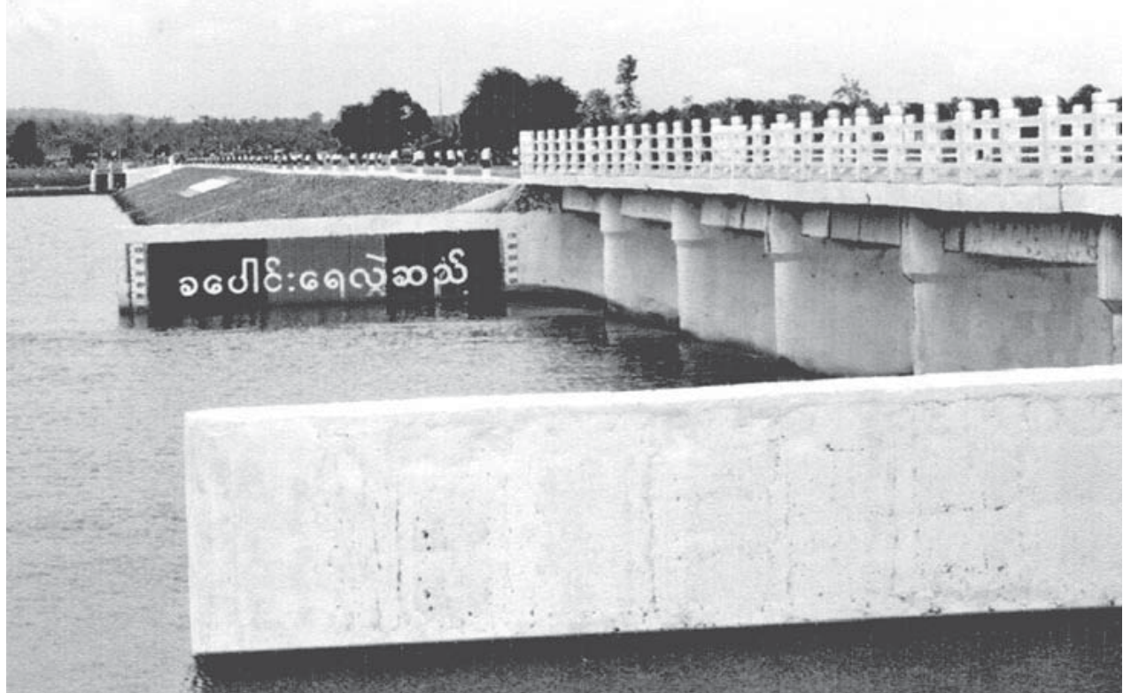
Khabaung Diversion Dam.
