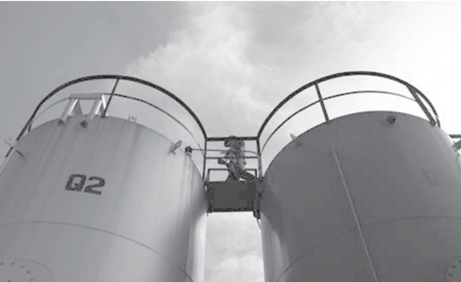
An employee of Petron Corp, the Philippines’ largest oil refiner, walks between blending fuel tanks at the Pandacan oil depot in Manila, on 18 June, 2008. Crude prices rose slightly Wednesday after a US government report showed a massive increase in crude stockpiles last week. —XINHUA
