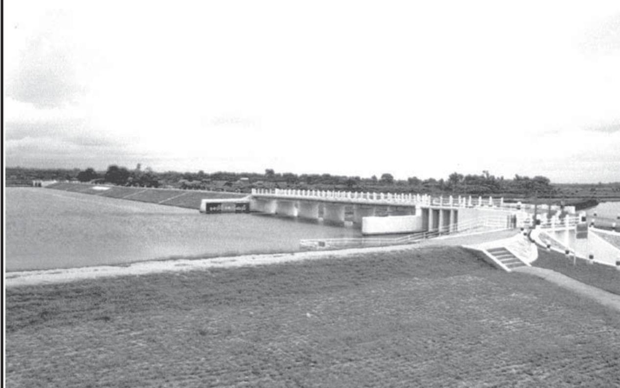
Water being stored at Khabaung Diversion Dam.
