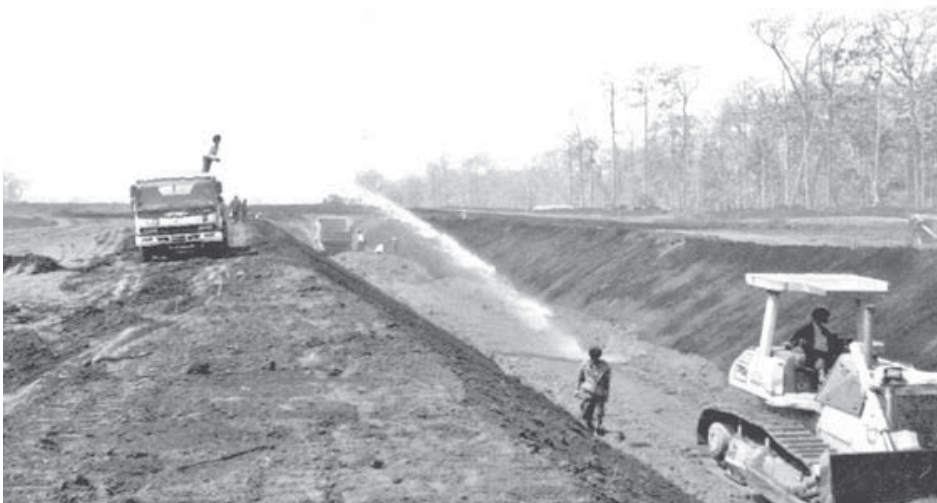
Earth work of the embankment and lower structure of Kengkham Dam is under construction with the use of heavy machinery.
