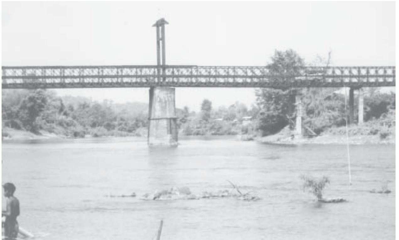
Photo shows existing Hsipaw Dokhtawady Bridge.
