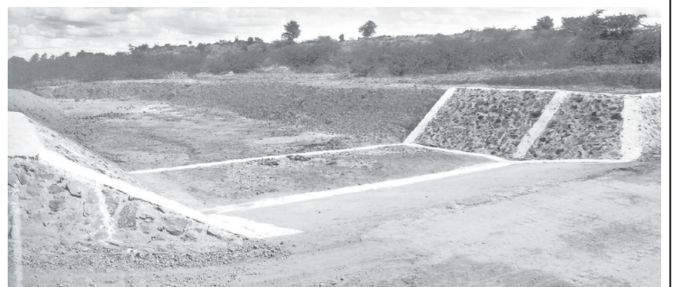
The 40-foot-wide spillway of Minkan Dam.
