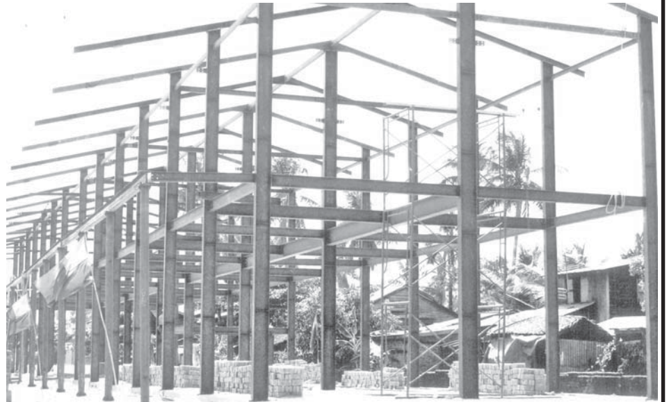
A school building under construction.
