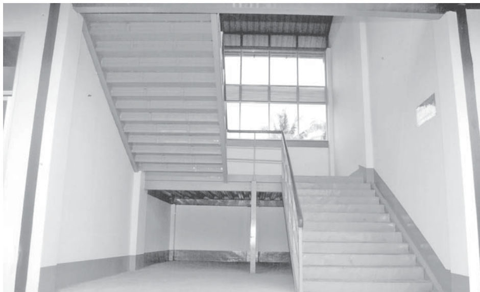
Staircase of school building constructed with steel structures.
