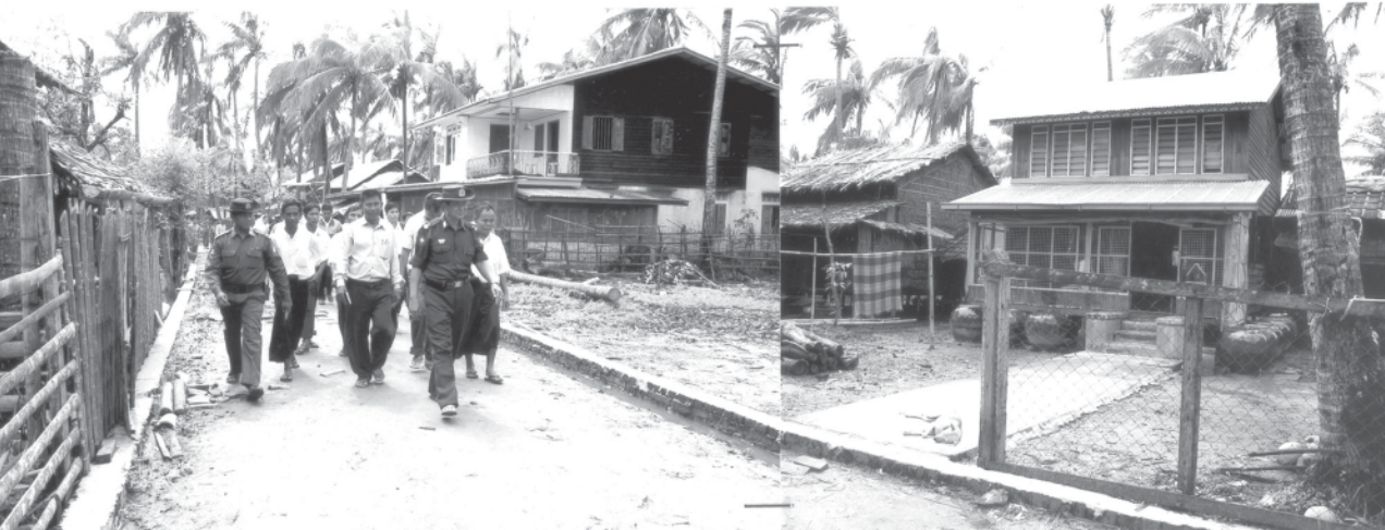
Minister Maj-Gen Aung Min inspects houses which have been repaired in Dedaye. —RAILWAYS
