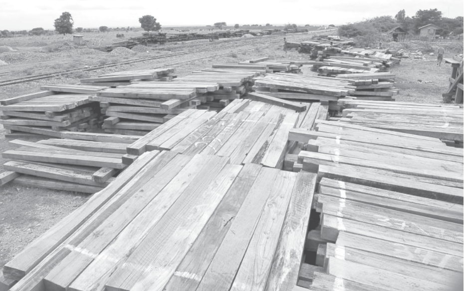
Sleepers to be used in constructing railroad.
