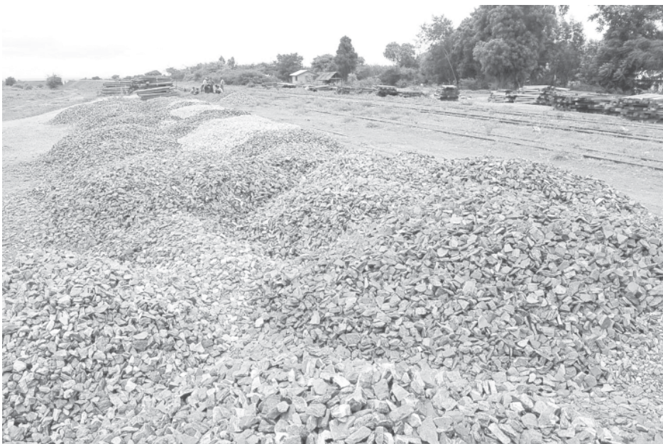
Track ballast are stockpiled to construct new railroad.
