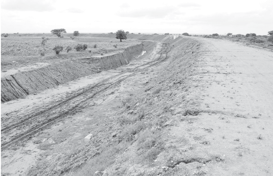
A construction site of railroad project.
