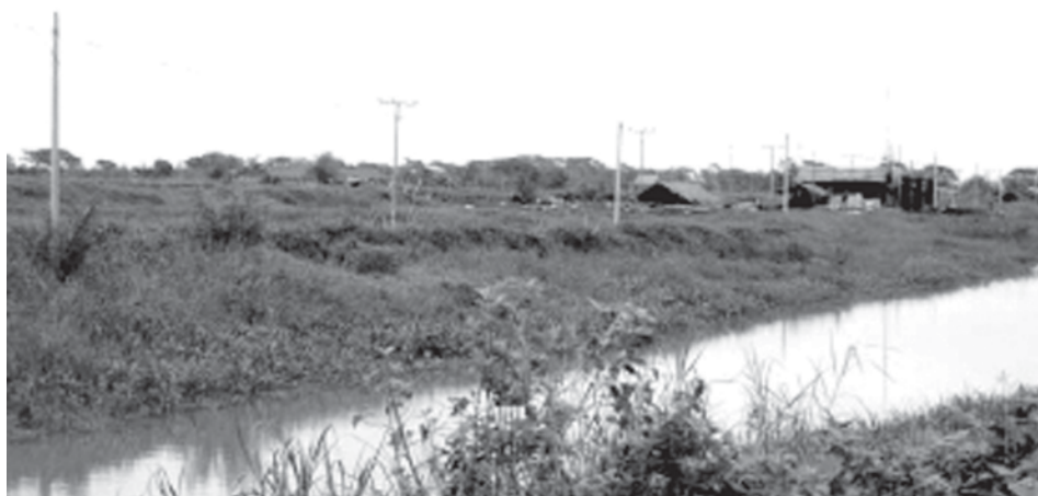
Completion of overhead fiber cable posts seen on Yangon-Maubin linkage on 23-5-2008.
