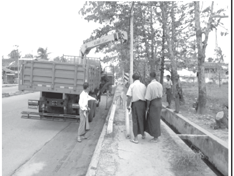
Telephone posts being re-erected in Hlinethaya Industrial Zone with the use of heavy machinery on 15-5-2008.
