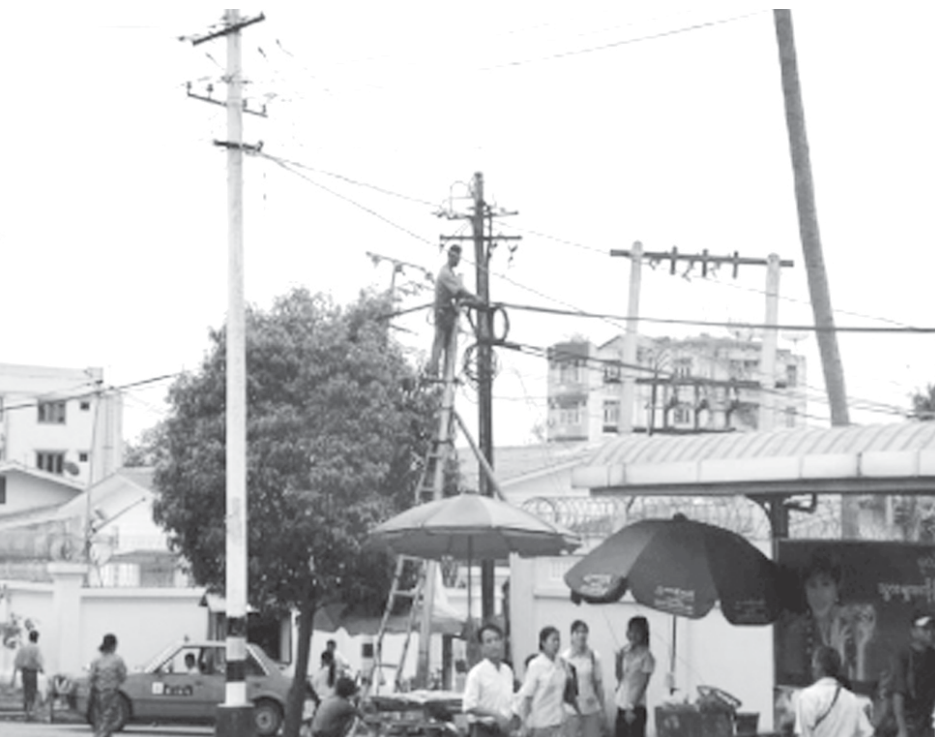
Workers repairing damaged cables in Mayangon area on 11-5-2008.
