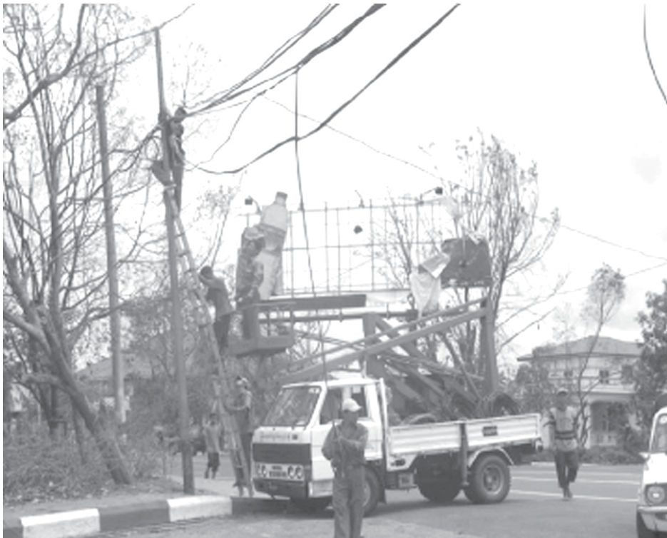
Workers repairing telephone post and cables in Maunghtawlay area on 13-5-2008.
