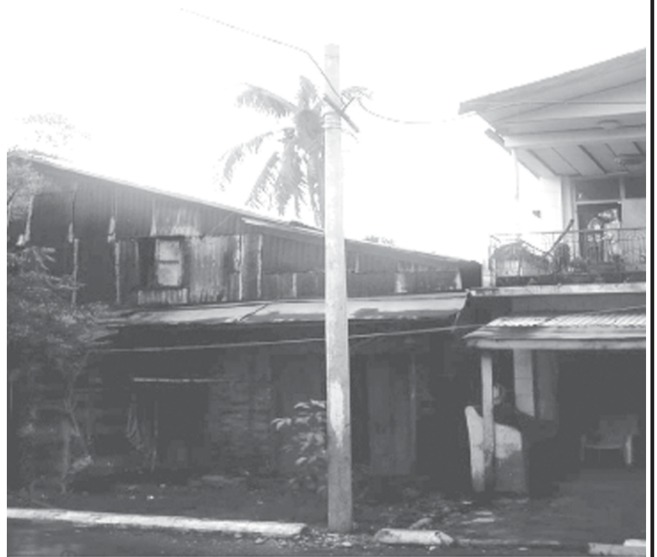
Substitution of new telephone post and installation of cables in Mawlamyinegyun on 13-6-2008.
