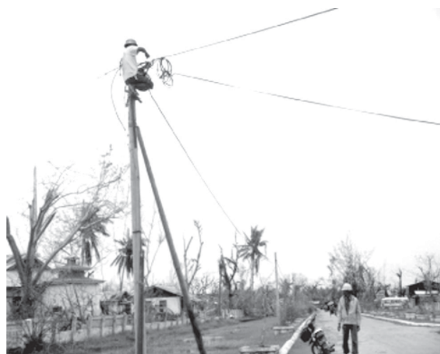
A worker linking cables in Pyapon on 12-6-2008.
