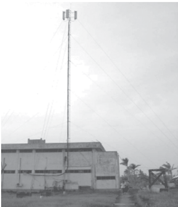
The photo shows the CDMA tower rebuilt in Pyapon on 24-5-2008.
