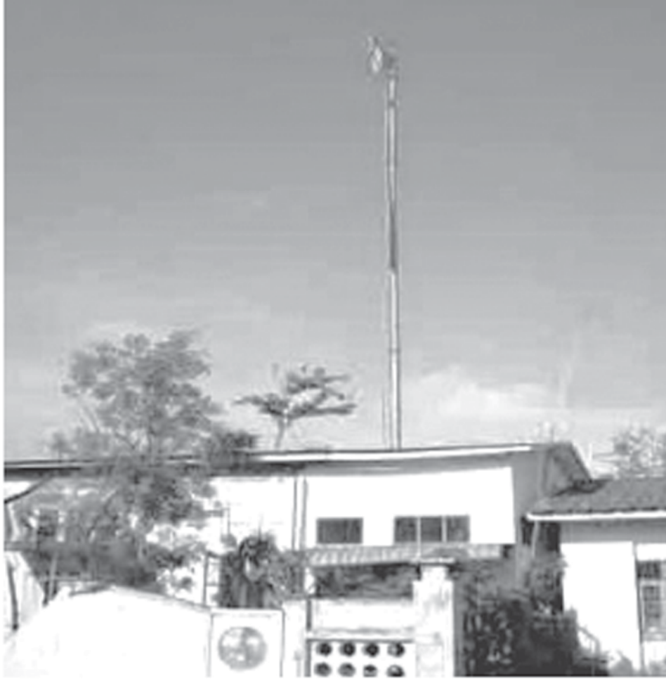
The photo shows renovated microwave building and tower in Mawlamyinegyun on 3-6-2008.
