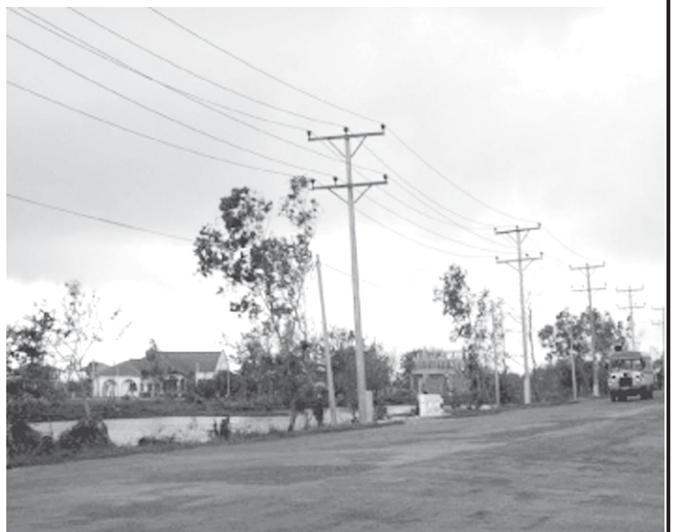
The completed overhead fiber cables on 20-5-2008.
