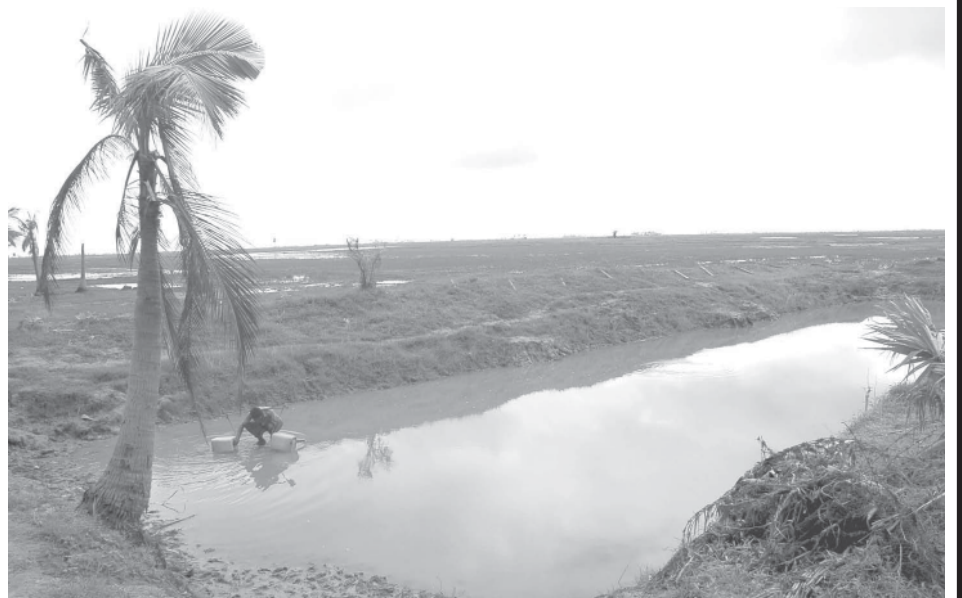
Local people can use fresh water from a lake that has been repaired in Thinganlay Village.
