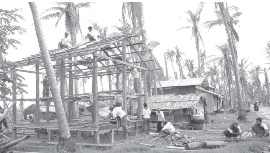
USDA member youths rebuilding ravaged houses hit by the storm in Thinganlay Village.
