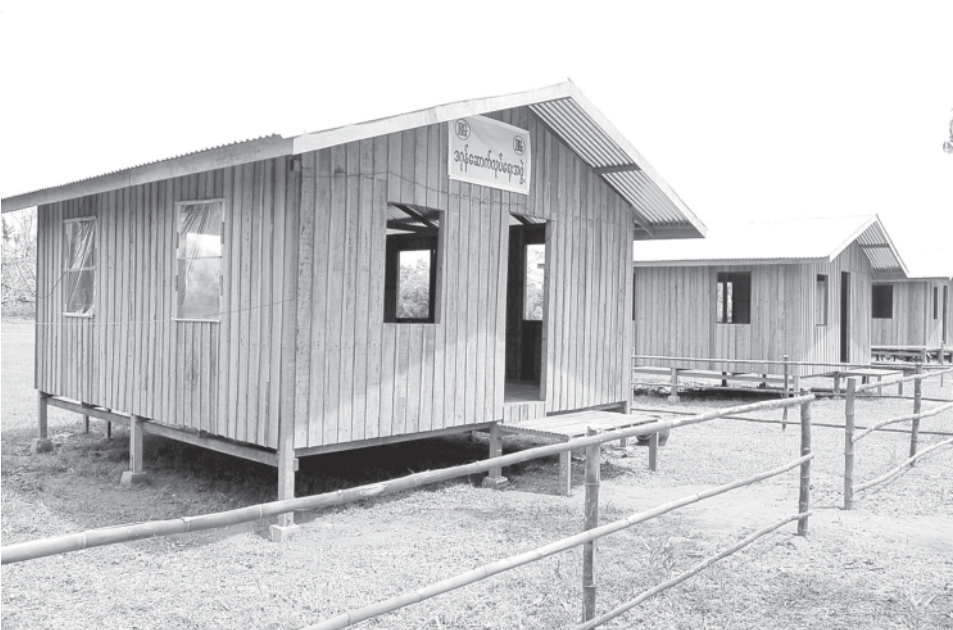
Homes for storm survivors seen in Kadonkani Village in Pyapon Township. President of CB Bank U Khin Maung Aye funded construction of the homes for the storm survivors.—MNA
