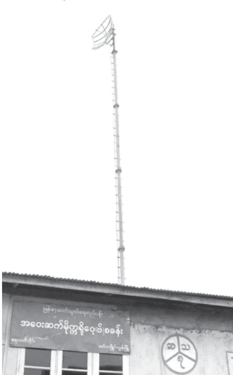
The temporary tower installed at Mawlamyinegyun Township Microwave Station.
