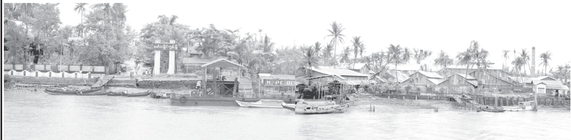
The photo shows progress in repairing houses and buildings in Mawlamyinegyun Township.
