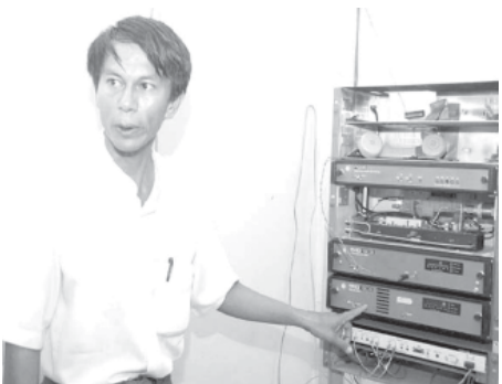
“CDMA telephone lines have been repaired 95 per cent.”
