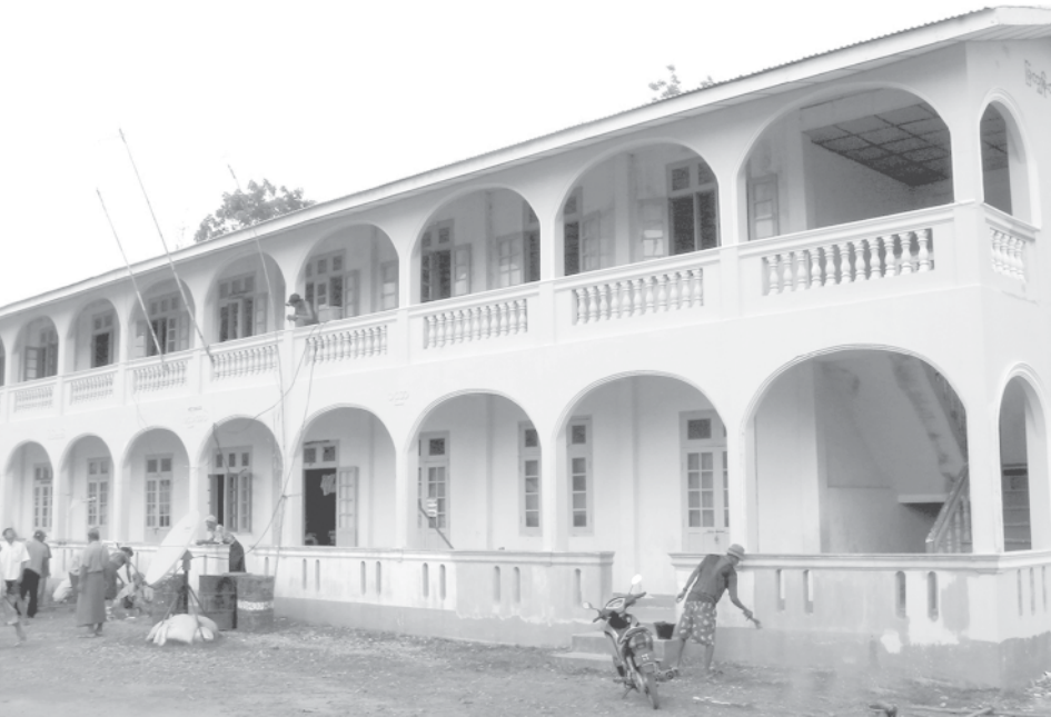
The repaired Hainggyikyun Basic Education High School.
