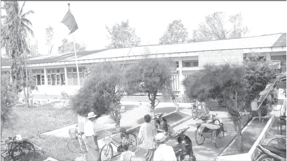
The photo shows the already-repaired Mawlamyinegyun Hospital.
