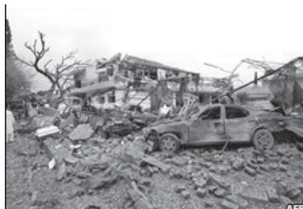
Damages seen after bomb blast.
